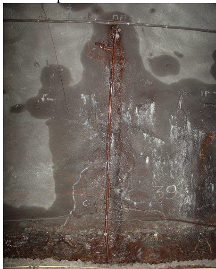
Figure 7: Drainage pipe at chainage km 1512+610, Nuolja 2004-10-07
