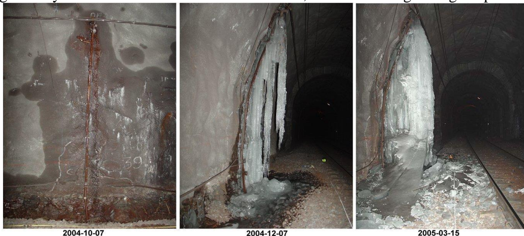
Figure 12: Drainage pipe, Nuolja chainage km 1512+610 left, at different inspections
