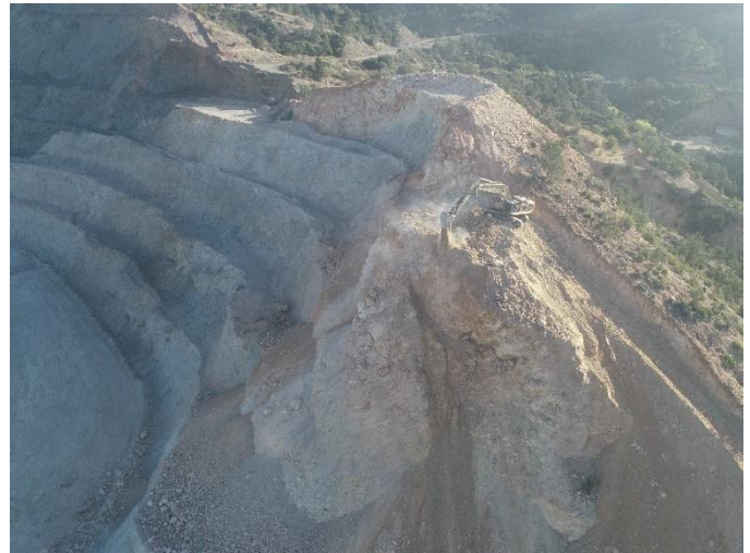
Fig. 1. Plan to excavate out remaining unstable ground
