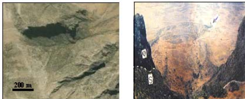
Fig.7: Left) Google Earth image facing south showing the crown area and side cliff of Qara Cahttan Landslide, Right) Photo from the crown area [3]
