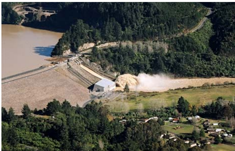
Figure 17: View of Matahina Dam [20]
