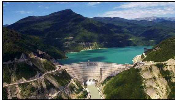
Figure 13: View of Enguri Dam, Georgia
