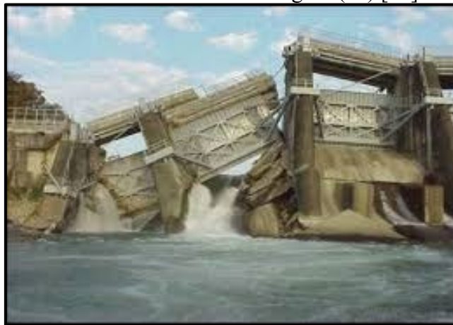
Figure 32: Shih Kang Dam gravity dam immediately after the Chi- Chi Earthquake on September 12th, 1999 [27].
