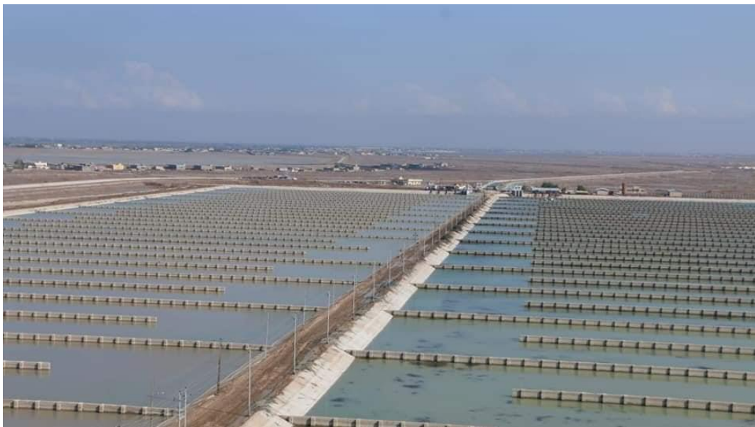
Figure 6: General view of R0 reservoir. (Source:[1]).
