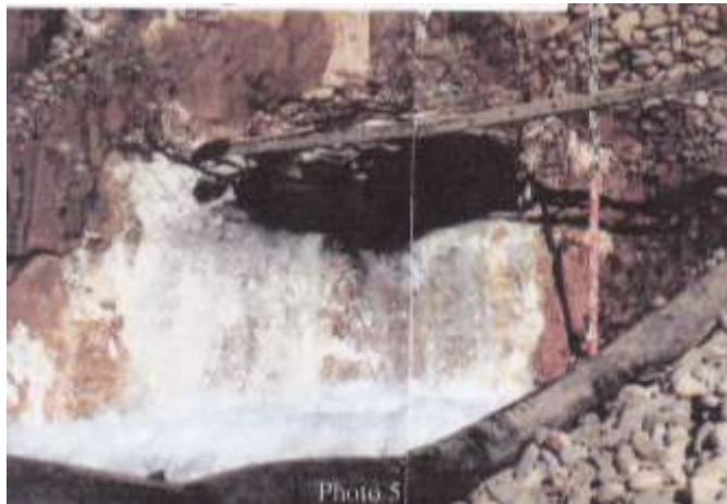
Figure 15: Flow (360 l/sec) from Underground aquifer into the intake/tailrace tunnel of the pump storage Scheme originating from Wadi Malih aquifer
