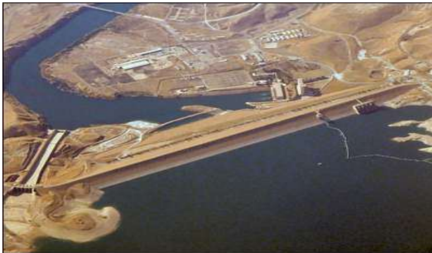
Figure 6: Aerial view of the Main Mosul Dam and appurtenant Structures
