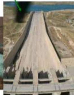
Site Photo 4. Close up of spillway (Photo courtesy of the USACE)
