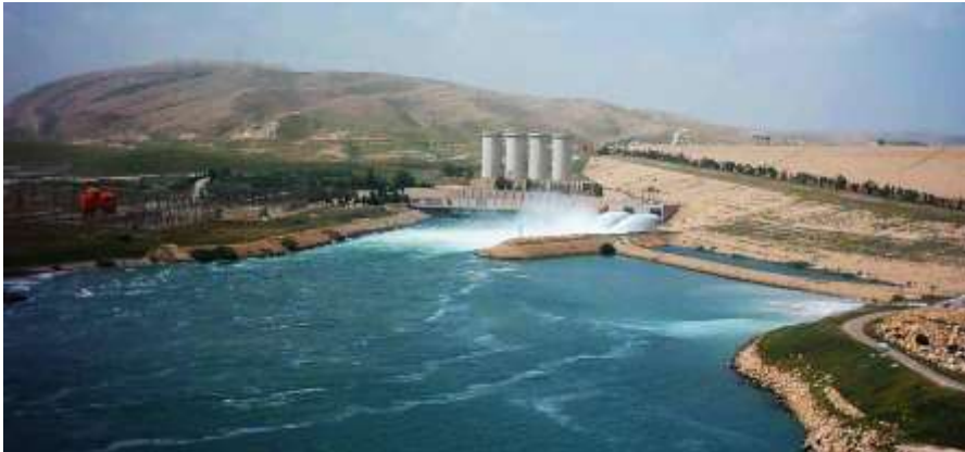
Figure 7: Downstream view of the Mosul Main dam Showing Bottom outlets and Power Station
