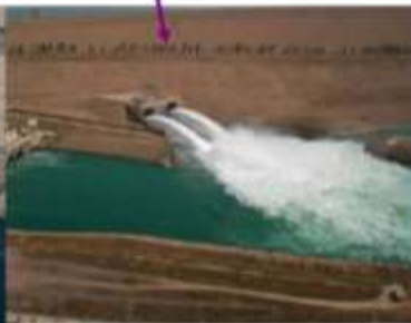
Site Photo 3. Close up of bottom outlet (Photo courtesy of the USACE)
