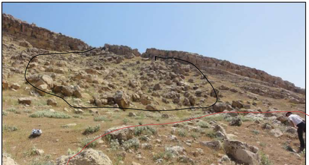
Fig.5: A small landslide (limited by black line) from the crown area of the main landslide. Note another very old slid mass (marked by red line)
