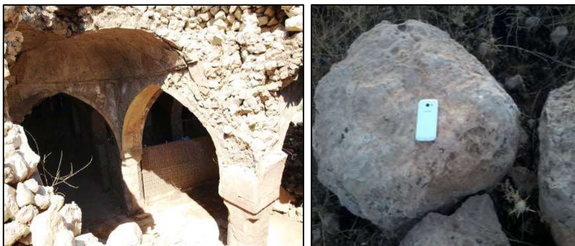
Fig. 7: Left) A collapsed old typical home in Alqosh town. Note the used rock in the building, all of them belong to the Pila Spi Formation. Right) A boulder derived from the Pila Spi Formation in the toe area; note the roundness of the boulder indicating long rolled distance and being very old; as a block
