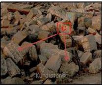
Figure 12: **Left**) A ruined Chaldean church, on Kirkuk's Citadel,note the pillarsare made of nodular and banded gypsum, **Right**) Banded gypsum blocks (**G**) used in ancient buildings, which are collapsed now.
