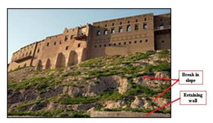
Figure 9: Houses built on the perimeter form a solid wall very similar to fortified citadels of medieval times. Note the recent break in the slopes due to cut of the slopes for road construction purposes, also note part of retaining wall in the lower left corner.
