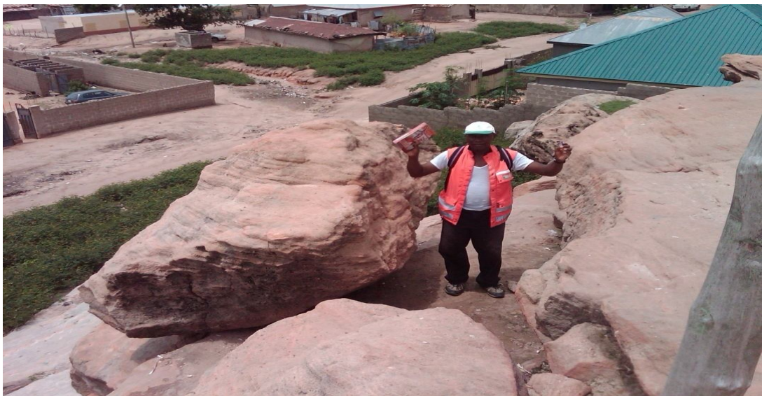
Photograph 3: Displaced boulders on hill slope puts buildings at the background at risk.
