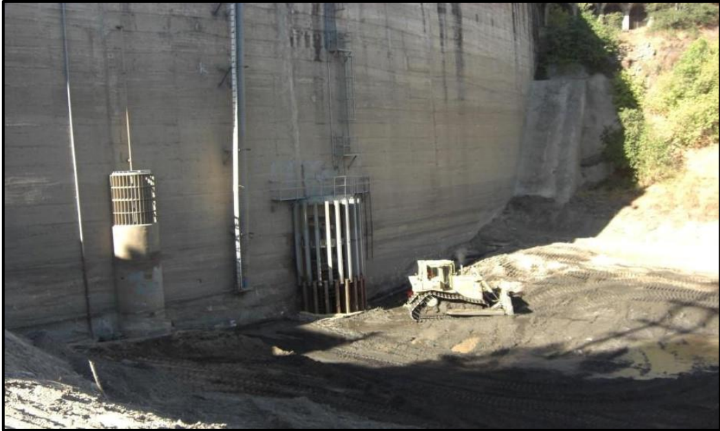
Figure 3: Intake Structure cleared pre- Station Fires of 2009 (Photograph dated on 8th June 2009 October 2010) [6].
