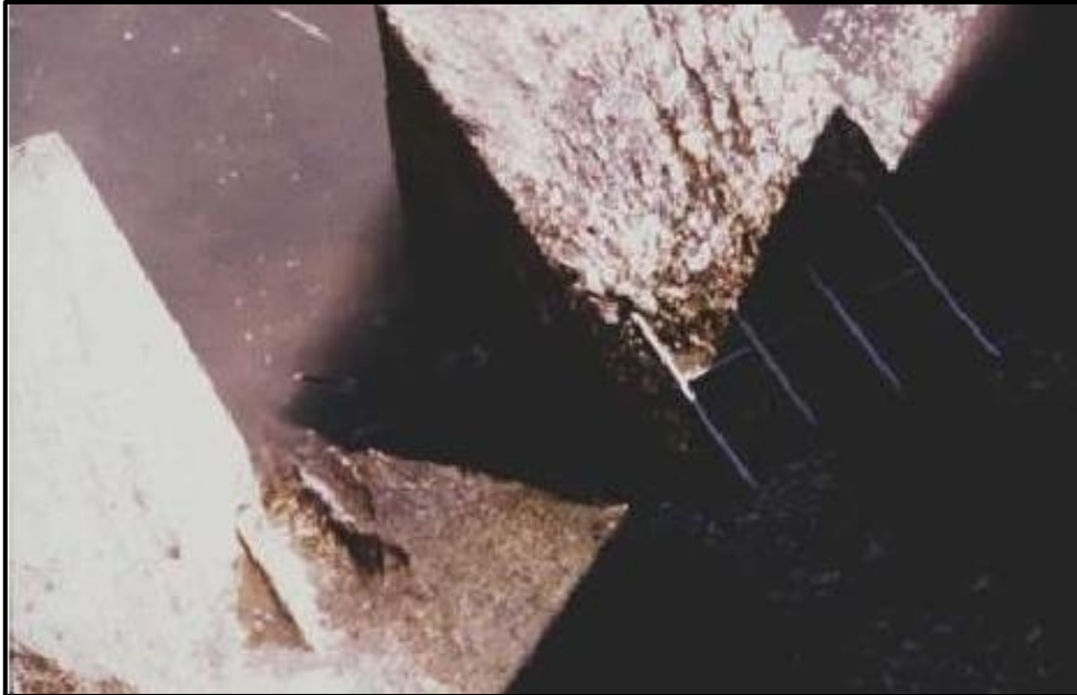
Figure 13: Close up photograph of sand abrasion of the Milburn Diversion Dam Spillway near Sargent, Nebraska [19].
