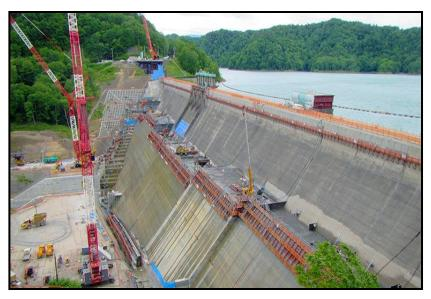
Figure 12: New Katsurazawa Dam during heightening operation in 2018 [24].
