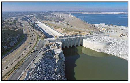
Figure 24: View of Folsom Dam Auxiliary Spillway after completion showing head works and chute [37].
