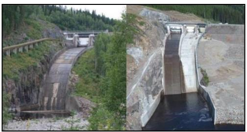
Figure 19: Höljes dam spillway: (Left) Original layout with two gated openings and a timber flume (Right) After refurbishment, with a 17m new gated opening added adjacent to the existing ones.
