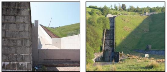
Figure 21: Usk Reservoir Dam Spillway views from downstream, after renovation (Left), before renovation (Right) (Photo by Mat Fascione) [32].
