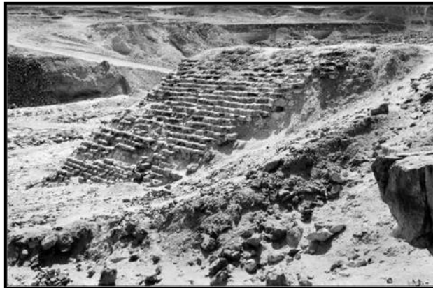
Figure 3: Remains of the Sadd el Kafara dam (about 2600BC), on the right bank of the wadi Garawi one of the oldest known large dam in history. View from upstream (photo of G.Albecht), [5].
