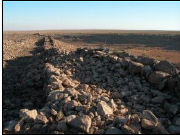
Figure 1: Remnants of Jawa Dam in Jordan [1].
