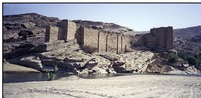
Figure 2a: Ruins of Marib Dam [4].
