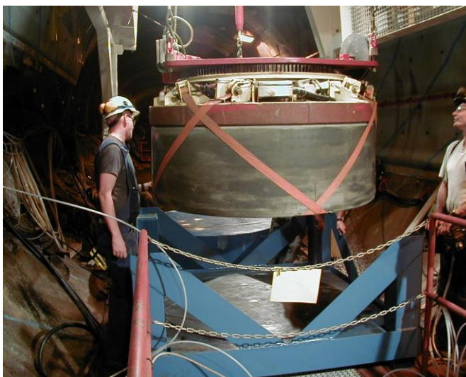
Figure 1: Placement of a 2000kg clay block with 1.80m diameter of smectite-rich clay (MX-80) being placed in a shallow deposition hole in SKB's ÅSPÖ underground laboratory (Photo: Ramqvist).
