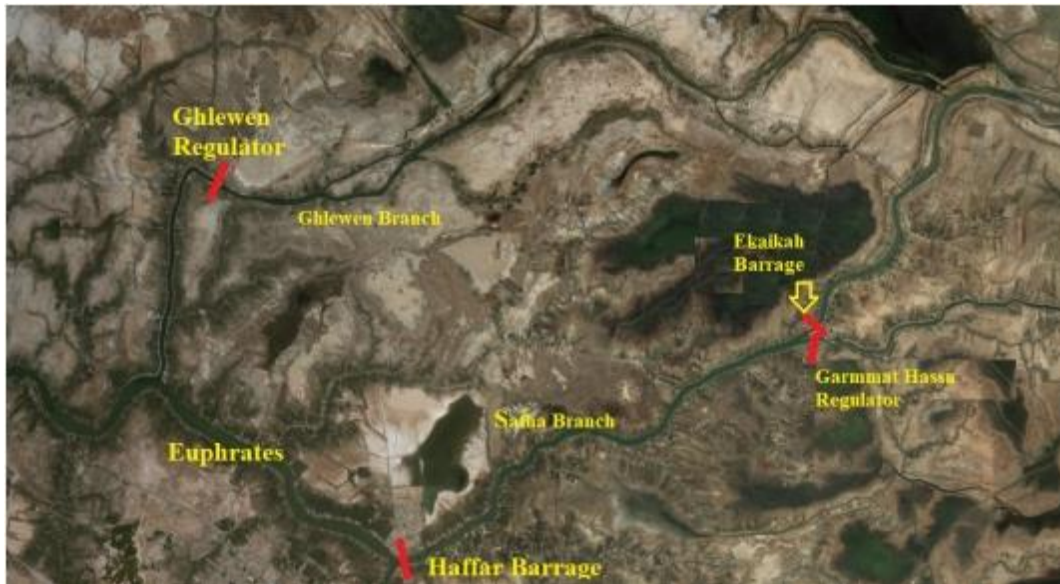
Figure 6: Main structures at Euphrates near Souq Al-Shouyokh. (Esri, 2019). (Edited by Author).
