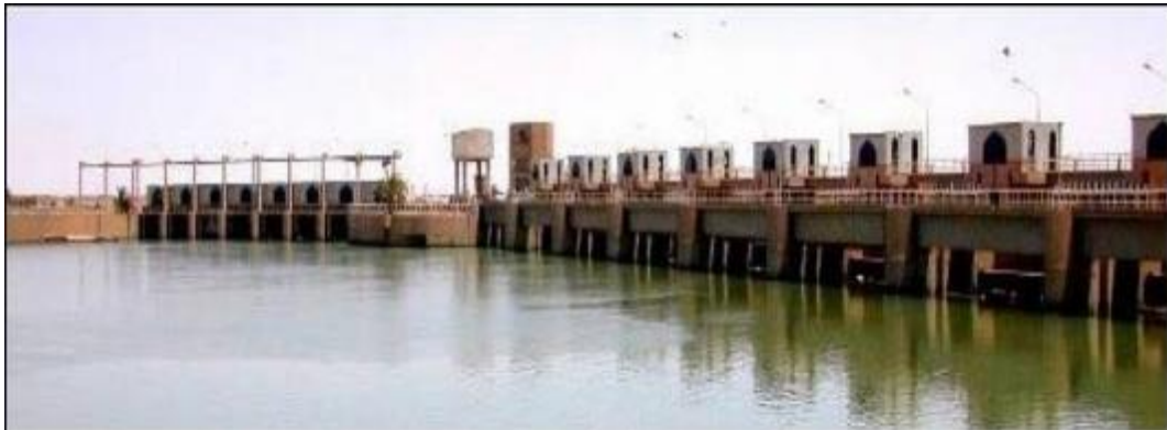
Figure 2: An upstream view of Fallujah Barrage and Combined Canal head regulator (Iraqi Ministry of Water Resources, 2019).
